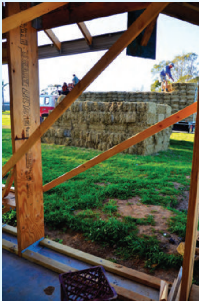
④ A delivery of bales of rice straw is unloaded. In the foreground are the frames they will fill. All case study photos by Tim Gould
