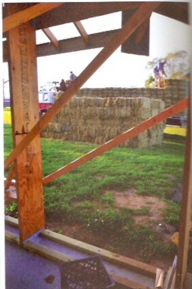
⑥ A delivery of bales of rice straw is unloaded. In the foreground are the frames they will fill. All case study photos by Tim Gould
