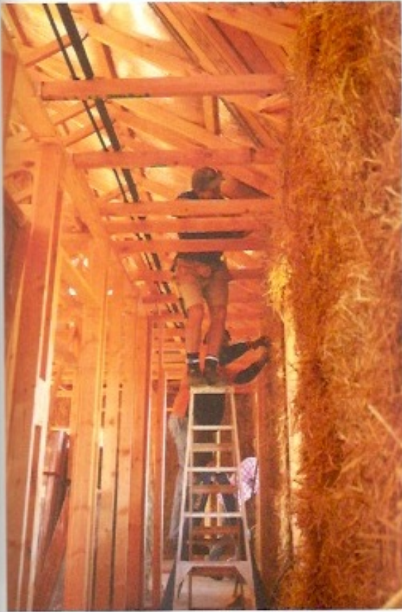
⑤ Volunteers work on installing the final layer of bales.
