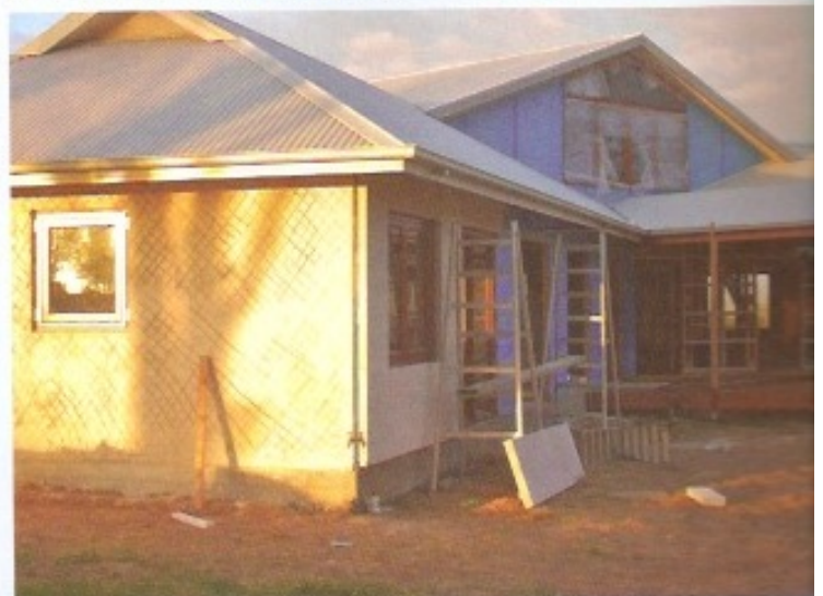
⑥ Once the straw bale walls are complete, the exterior is rendered with a lime mixture.
